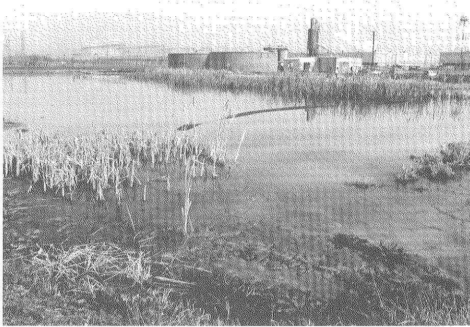
Containment lagoons (left) that once held hexavalent chromium sludge were one of four areas requiring environmental restoration identified by the U.S. Department of Energy at the Portsmouth Gaseous Diffusion Plant. The chromium, used to inhibit corrosion in the plant cooling water system, was replaced by a more environmentally acceptable phosphate-based corrosion inhibitor. A grassy field (right) now stands where chromium-laden sludge once stood in the containment lagoons.
