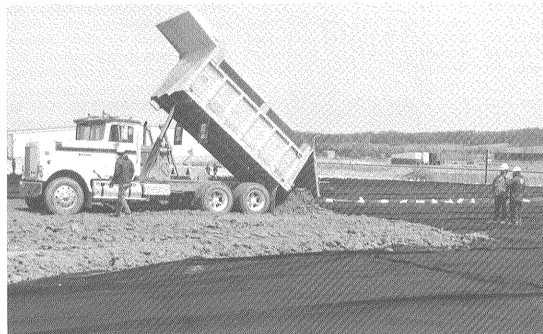
Soil was taken from another area of the plant and moved by more than 10,000 dump truck trips to this covered former low-level radioactive landfill at the south end of the plant (below).
